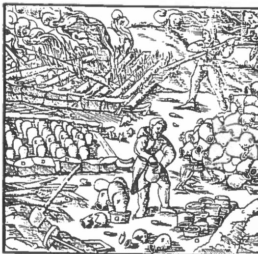
Figure 15. Smelting mercury ore, from Agricola's *De Re Metallica*. Mercury was relatively easy to procure — just heat the ore.
